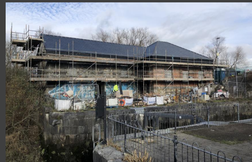
Salvaged Bricks to Canal Harbour Building
