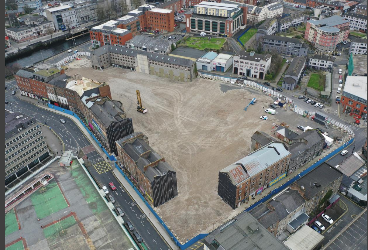
Dec 2022 - Site cleared and enabling works 100% complete
