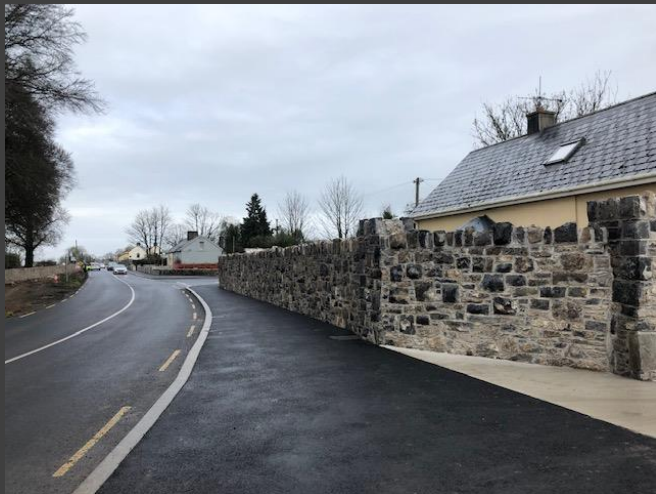
Re-use of Stone in Herbertstown Cemetery Wall Construction
