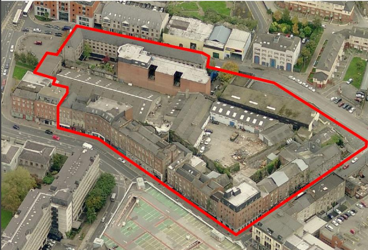
Dec 2020 - Site at commencement
