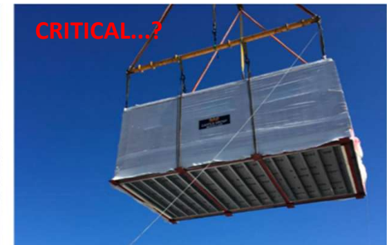
Figure 2: Module being hoisted with specially designed lifting frame
