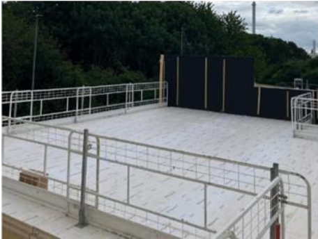
MOISTURE MONITORING FROM FACTORY TO SITE
