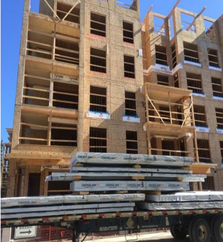
PRE-APPLIED TIMBER PORTECTION FORM MANUFACTURE TO SITE
