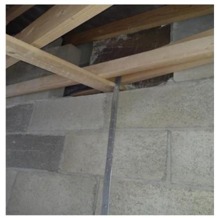
Blockwork removed from inner leaf of gable wall to accommodate roof truss
