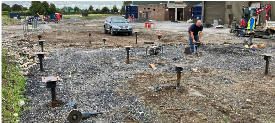
Removal of topsoil (no foundation trenches required), install screw piles
