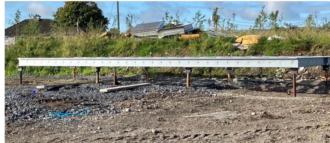
Install pile caps (either steel or concrete), and fit prefabricated cassette
