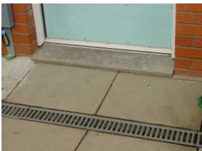
Figure 9 Typical proprietary drainage channel located on the external landing
