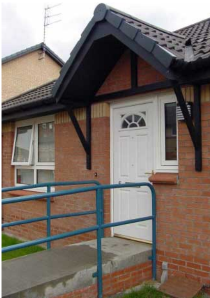
Figure 2 Additional features on the external landing in the form of a porch to give weather protection and railings to give support
