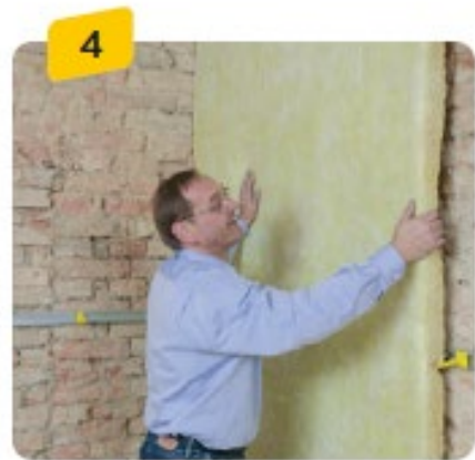
Hang Insulation on plastic clips
