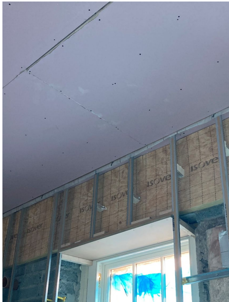
Fire rated ceiling
