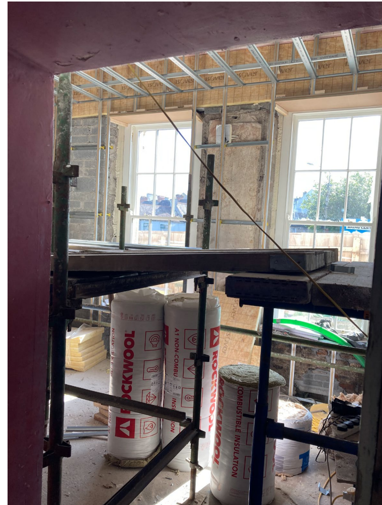
Rail system for final layer of plaster board
