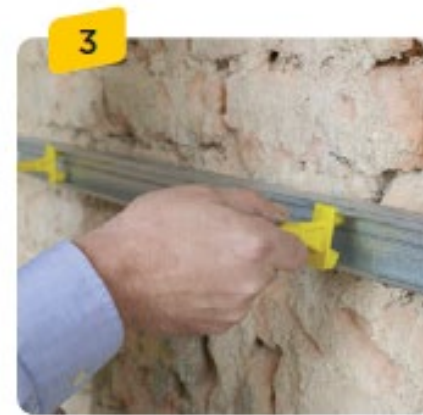
Fix plastic clip on horizontal C-channel
