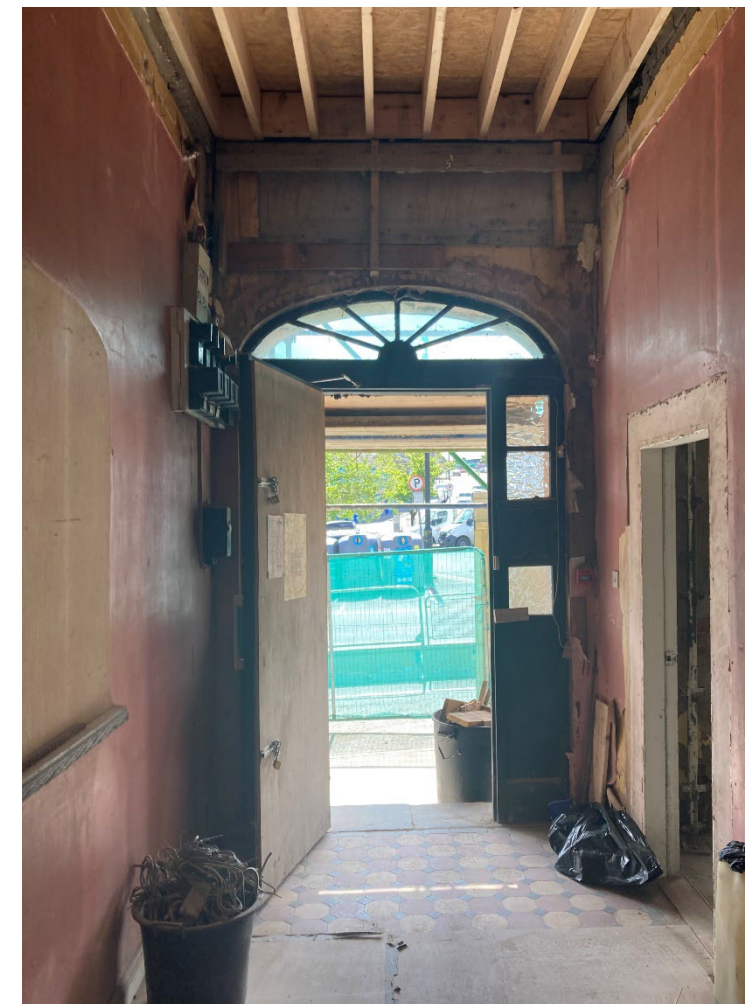
New floor joist required.
