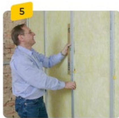
Fix plastic clip on vertical C-channel, adjust until plumb and lock in place
