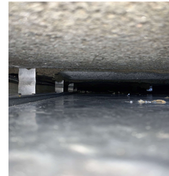
Cavity barrier at eaves
