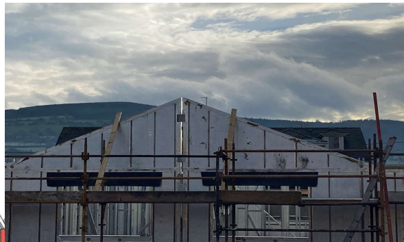
Cavity maintained at party walls
