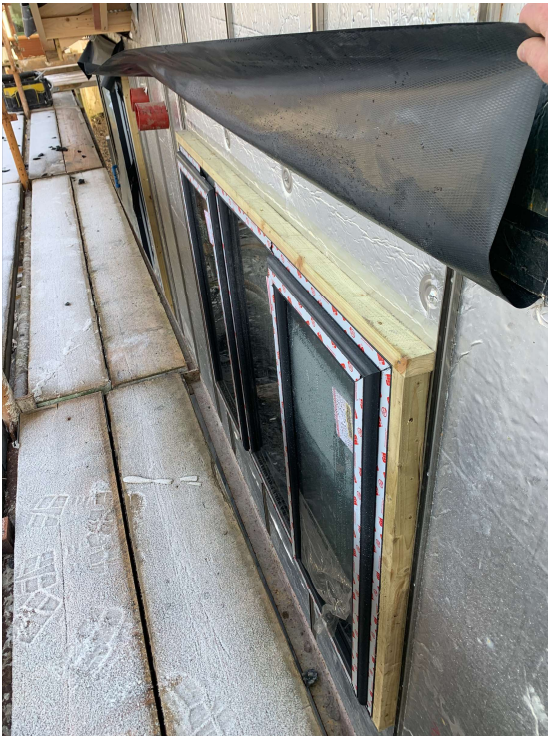
Cavity barrier at window
