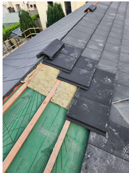
Fire stop roof cavity at party walls
