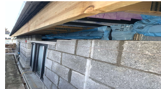
Cavity barrier at eaves
