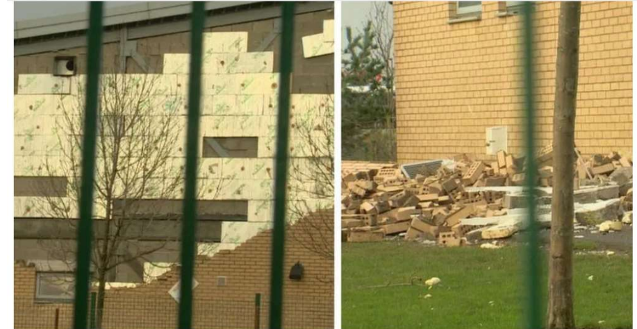
The problems first became apparent when engineers examined the wall that collapsed at Oxgangs Primary during stormy weather
