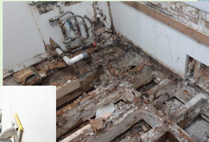
long term consequences of trapped water
