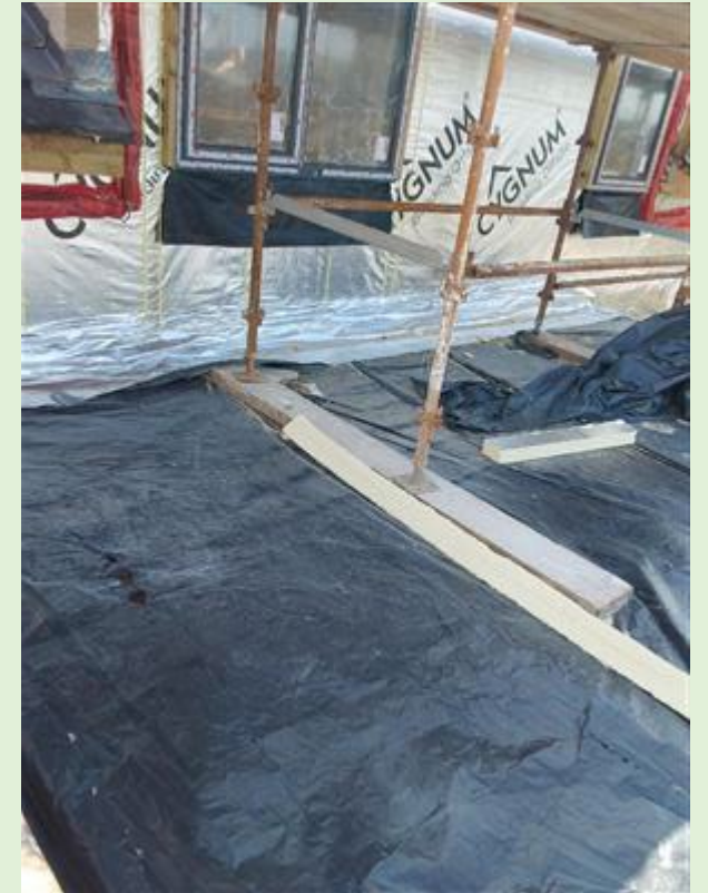
Temporary protection of elements not designed to be exposed long term such as timber roof decks
