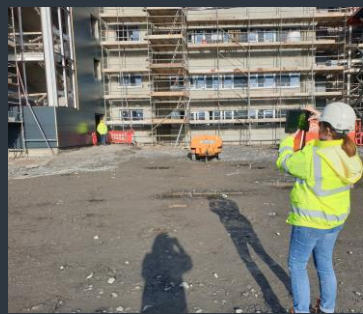
Donegal Building Control Officer, Donna Butler inspecting to ensure compliant buildings.
